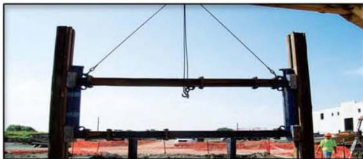
Above: The strut cart unit supported the slide rail system on the inside.
